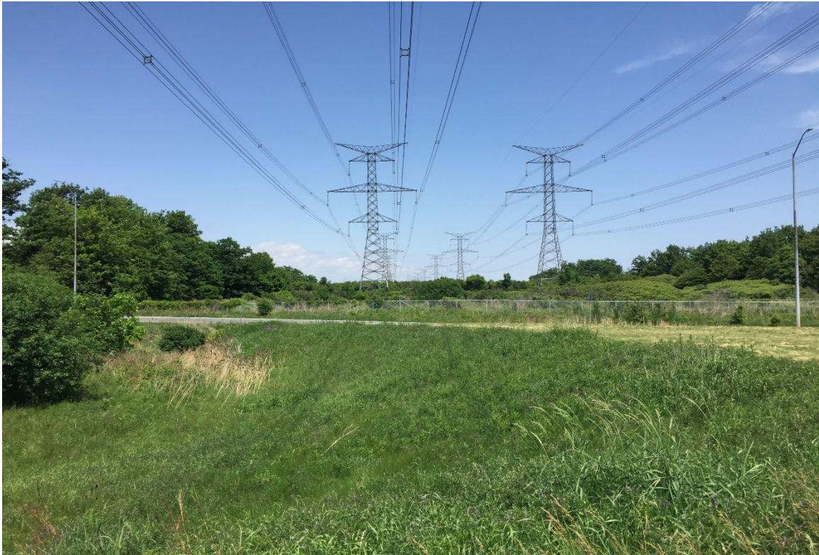
Photograph #33: View looking east from Mavis Road along the south side of the 407 ETR. The proposed runningway is to be located through these vacant/wooded lands and utility corridors.
