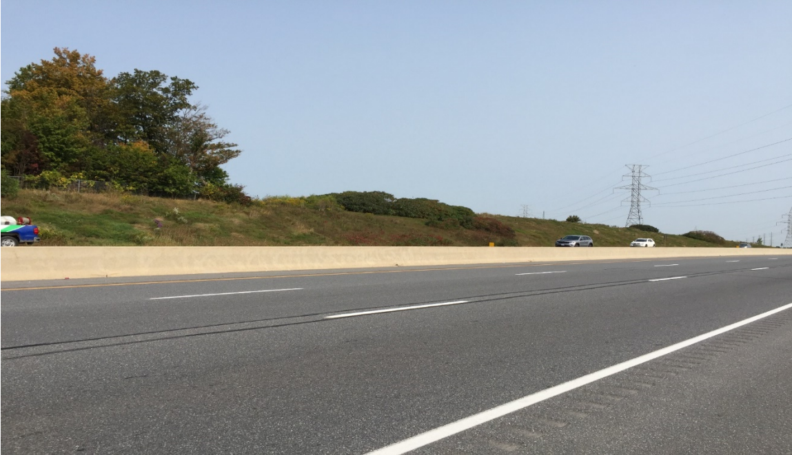
Photograph #6: View looking east along the 407 ETR showing the landscape the north runningway passes through, east of the Bronte Creek valleylands.
