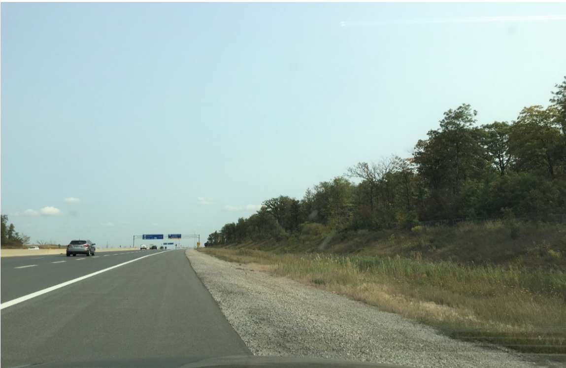
Photograph #13: View looking east along the south side of the 407 ETR, approaching Trafalgar Road, along the proposed runningway route.
