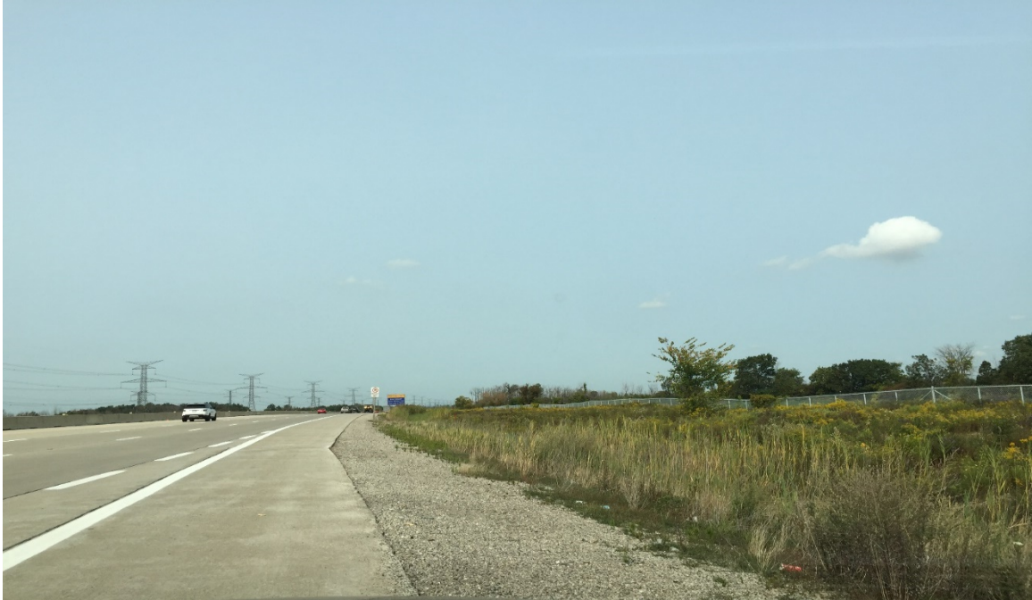
Photograph #17: View looking north along the 407 ETR corridor, just south of Eglinton Avenue at the approximate location where the runningway will cross from the west to the east side of the highway.
