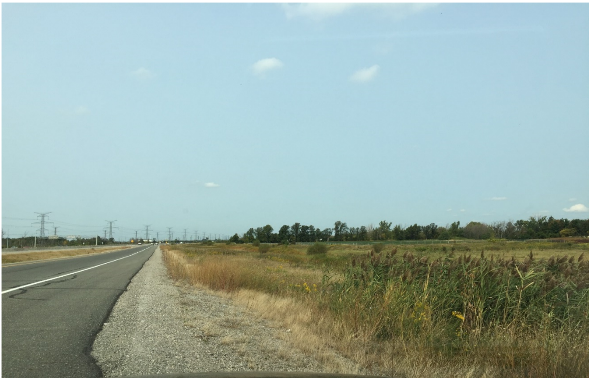
Photograph #23: View looking north along the east side of the 407 ETR corridor. The runningway will pass through these vacant lands.
