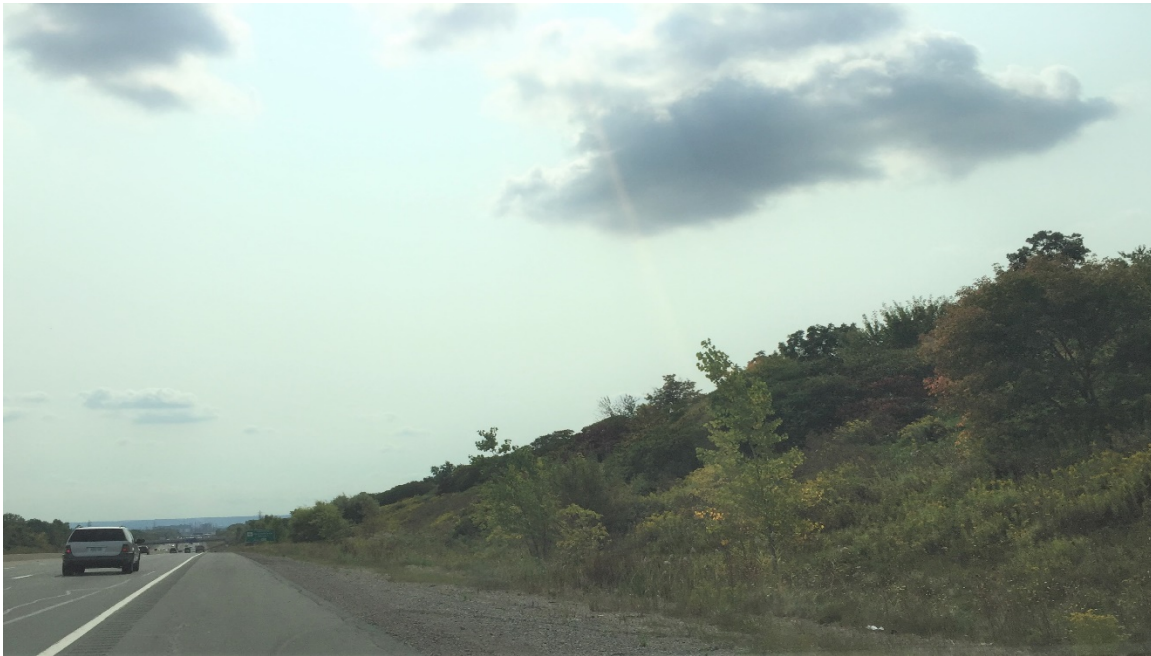
Photograph #1: View of the north side of 407 ETR, looking west down the proposed runningway corridor.
