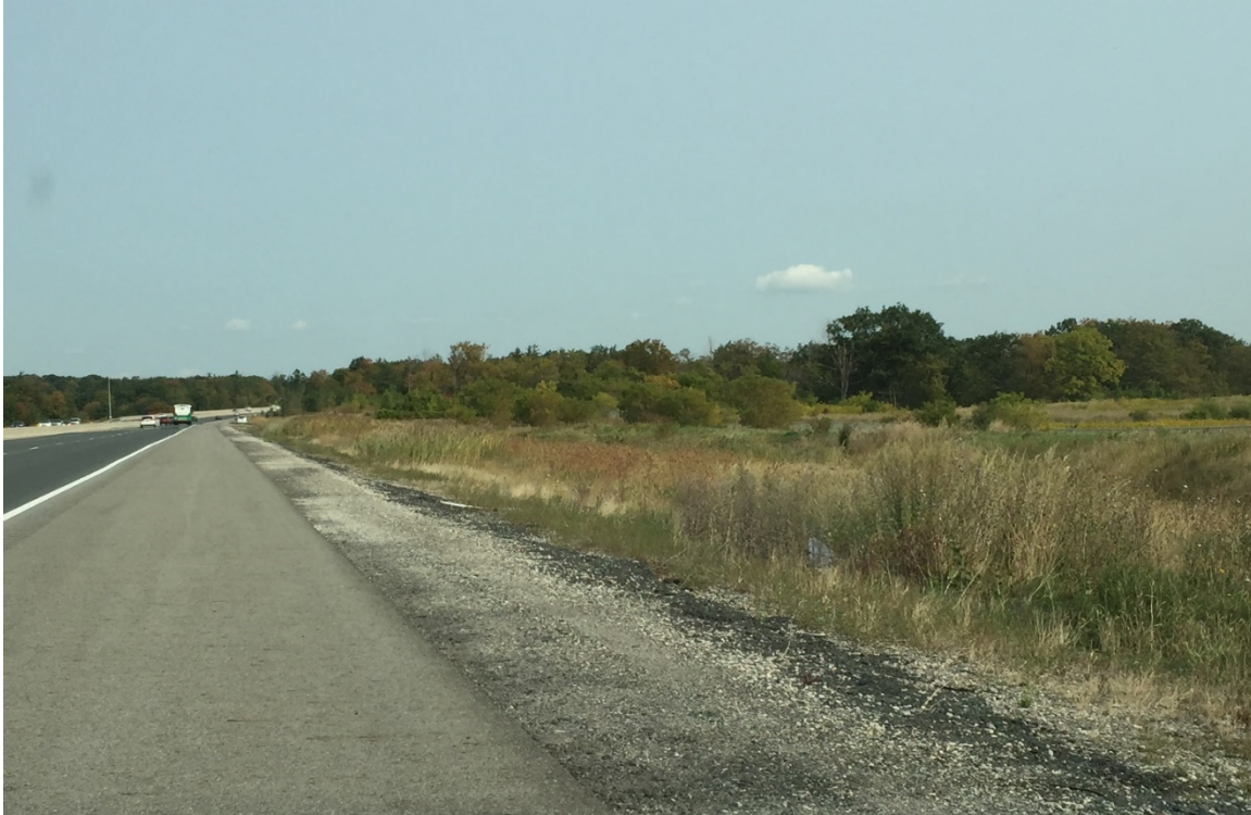
Photograph #9: View looking east along the south side of the 407 ETR, approaching the Sixteen Mile Creek valleylands.
