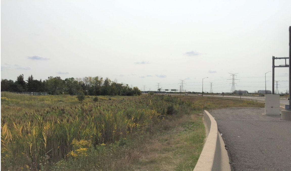
Photograph #24: View looking south along the east side of the 407 ETR corridor. From Derry Road. The runningway will pass through these vacant lands adjacent to the stream channel located in the foreground.
