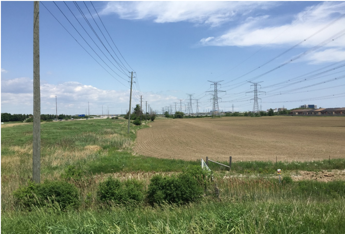
Photograph #36: View looking east from McLaughlin Road along the south side of the 407 ETR. This section of the runningway will terminate in the distance, beyond the Flecher's Creek valleylands. A residential development is located along the south side of the utility corridor.
